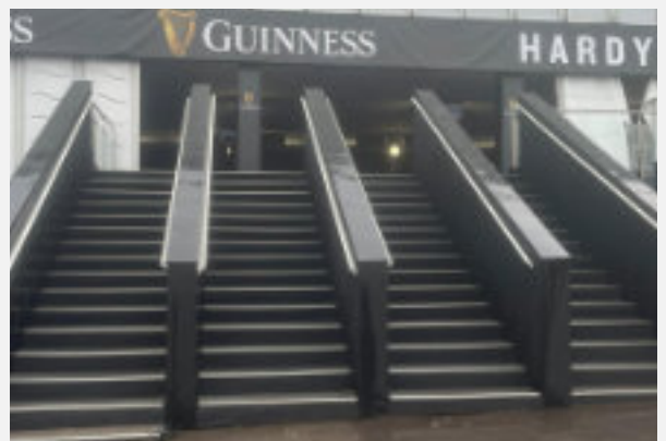
HOARDING FOR TEMPORARY STAIRCASE CHELTENHAM
