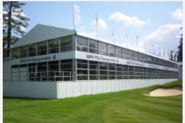
SUB-STRUCTURE HOARDING FOR PGA CHAMPIONSHIP
